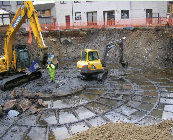
Figure 1 Excavation of contaminated soil from a gasworks holder tank located in a residential setting (courtesy of VHE Construction Plc).
